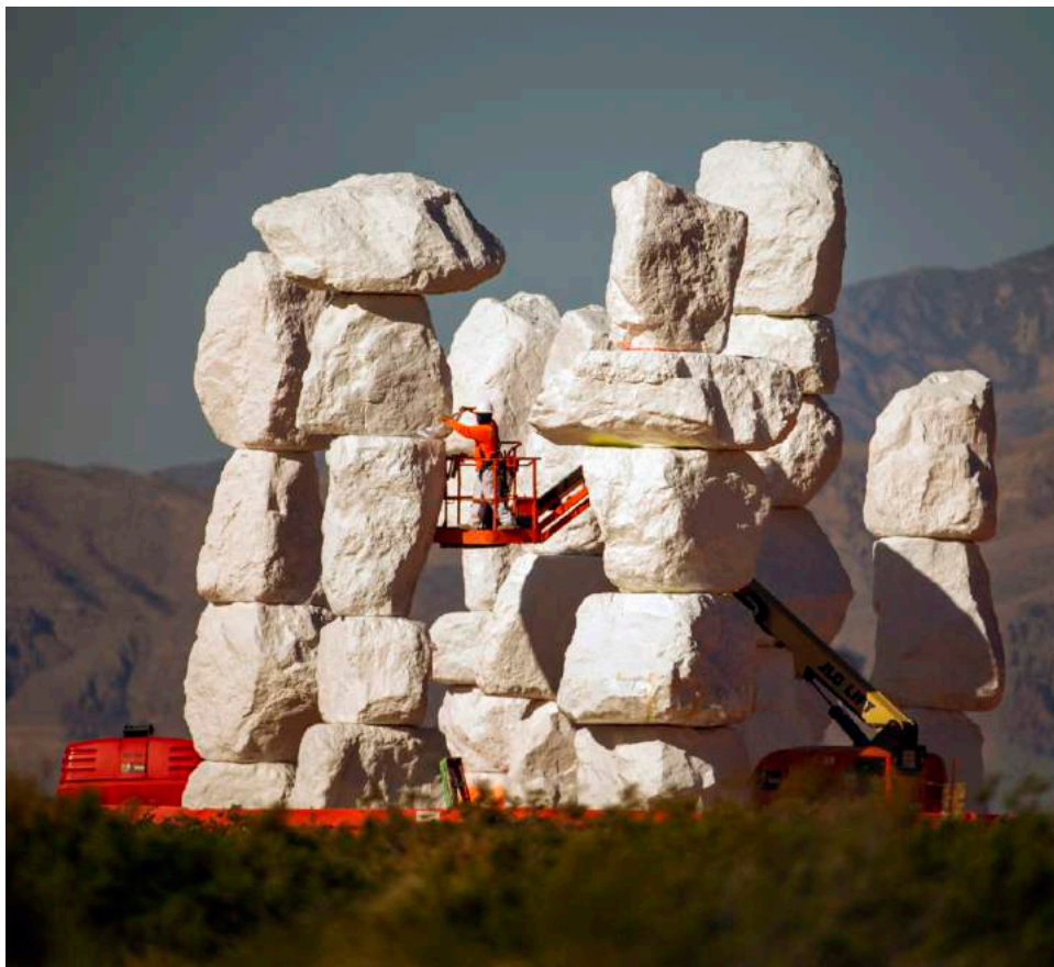
Ivan Ibarra applies primer on June 4. The towers stand 30-35 feet tall.
