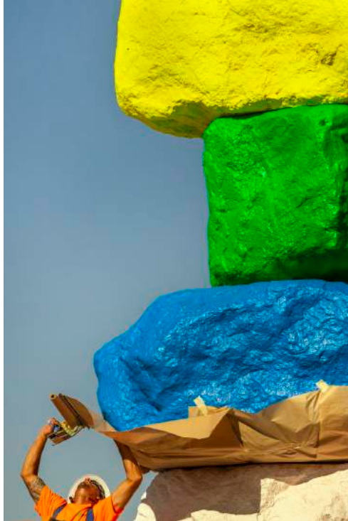
John Henderson masks off rocks to prevent overspray on June 14. Each limestone rock received between 10-13 coats of the same kind of paint used on cars.
